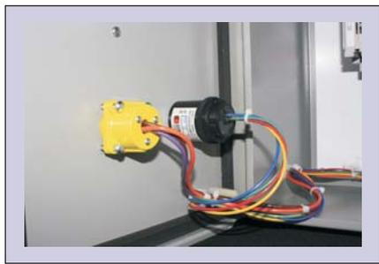
**Permanent Electrical Safety Devices (PESDs)** are defined as external devices permanently mounted to electrical systems that, directly or indirectly, reduce the risk of arc flash and/or shock hazard by providing feedback on the voltage state within the enclosure and eliminating proximate exposure to that same voltage. PESD combo units include voltage portals and voltage indicators.
