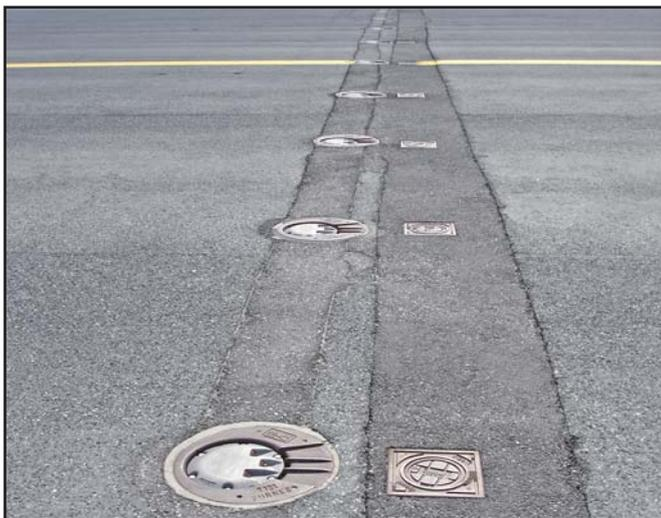
Full flush approach lights type SLAP in a base with straight edge installed at a Norwegian airport.
