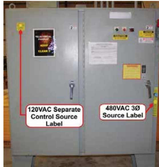
Fig.1 Voltage Source Labeling
