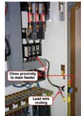
Fig. 6 Proper location of a three-phase portal
