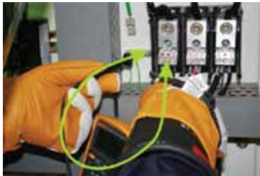
Fig. 4 Verifying the presence of voltage with a digital meter
