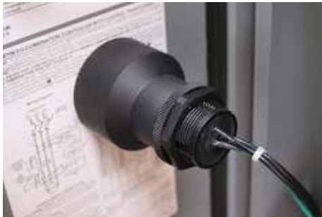
Voltage indicator with Bezel kit – back
